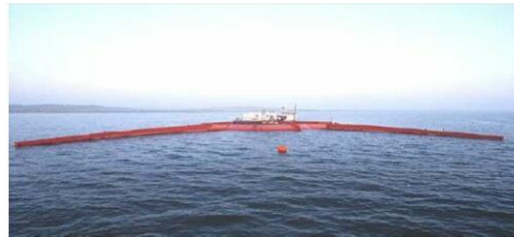
Image of wave dragon overtopping device
